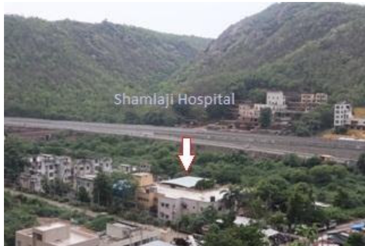
Aerial View of the Shamlaji Hospital Campus in the Valley of Aravalli Mountains Range
